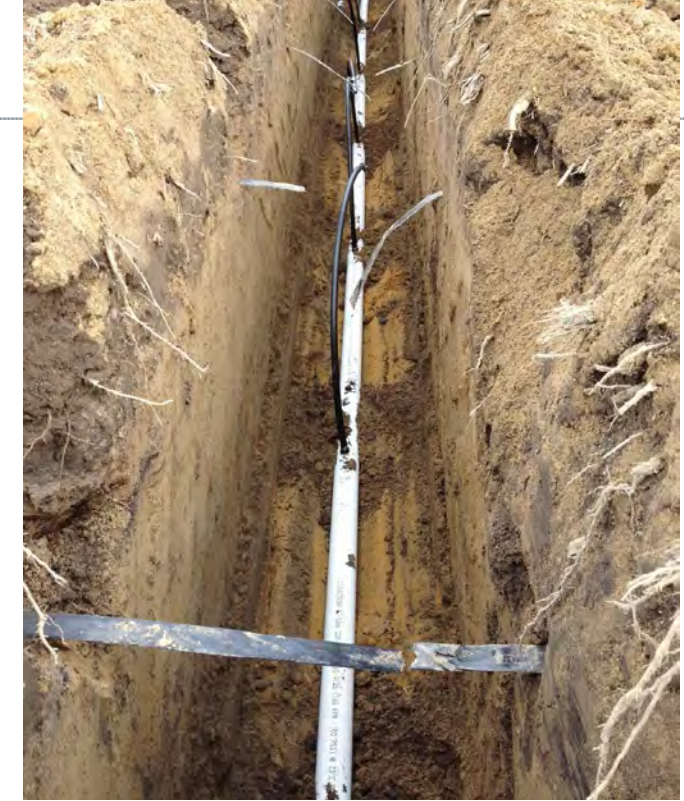
The irrigation drip tape is buried 14 inches deep on 44-inch spacings. A Magnum tractor equipped with the AFS Pro 700 display provided the RTK autoguidance and mapping. The excavation photo shows the main line with rigid risers hooking to the dripper lines. Boughner and Hill show a completed field, with risers in place to take in water pumped from a nearby pond.
